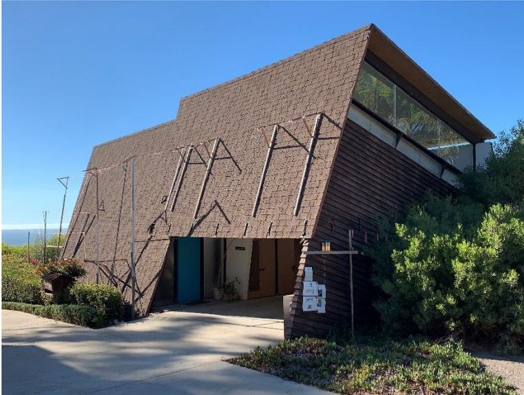
**Photo 2** Southeast corner detail, wood siding, fixed (top) and louvred (below) clerestory windows, view northwest
