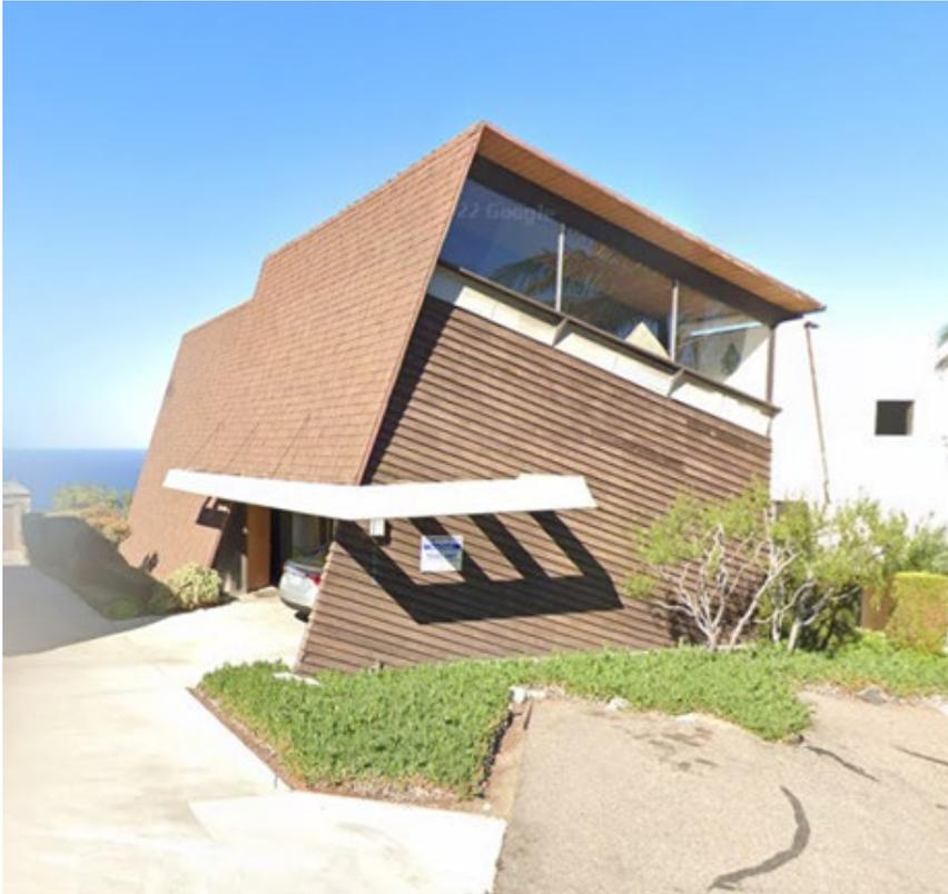
**Figure 2** House at 981 Summit Drive, Laguna Beach, completed 1961, Bud Evenson, designer; 2022; courtesy Google; note the distinctive, hyperbolic paraboloid carport roof form suspended from canted, paired masts and use of natural, stained wood
